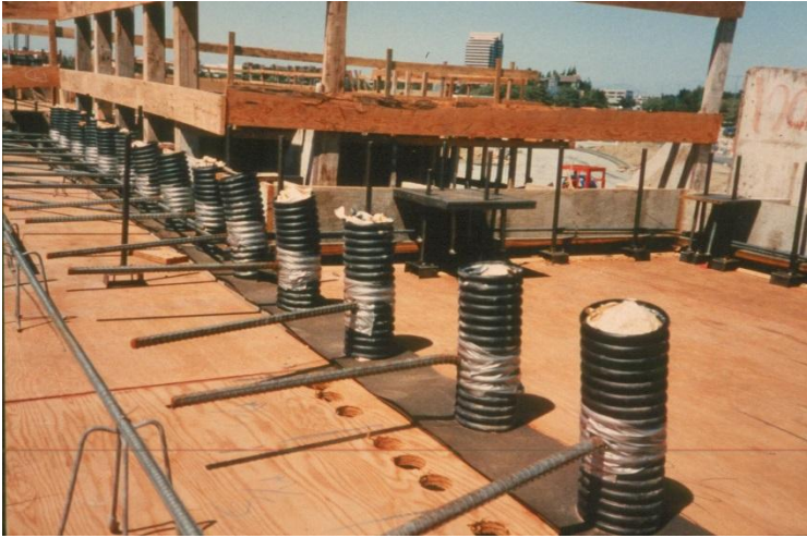
(a) Dowels extend into slab (P766)
