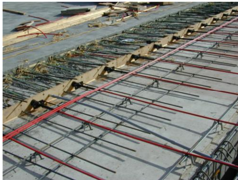
(a) Delay strip after concrete on one side is cast (P762)
