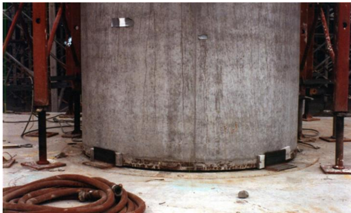
(a) Column base on slip pad (P767)
