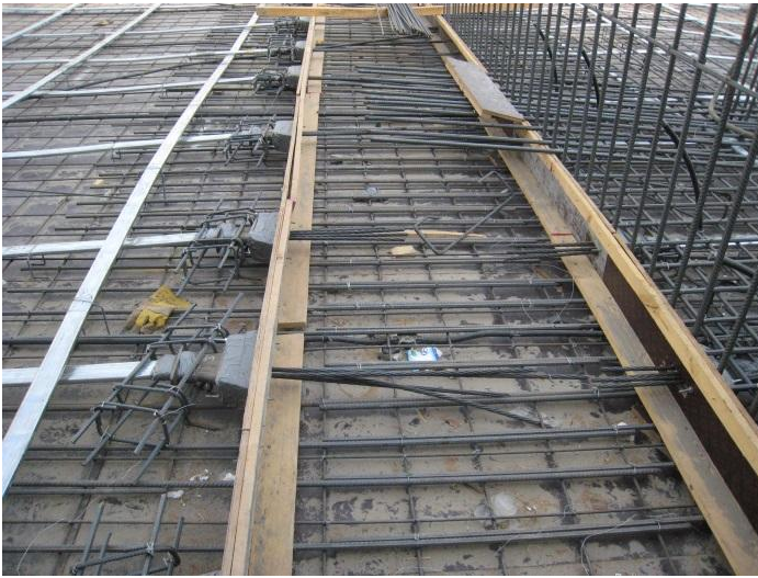
(a) Delay strip in preparation using grouted tendons (P746)
